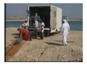
STS, have successfully completed the longest CCTV survey in the world utilising specific technology that was developed by us. The inspection of the 10 km, 24" drinking water main from Jebel Dhana to Sir Baniyas island represented a world record. Our professional services resulted in the local authorities issuing a second contract where we surveyed the existing 20" line running parallel to the new one. Both projects were completed well within the specified time and within the projects budget.
